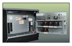
Circuits can be easily added or removed as your load requirements change
